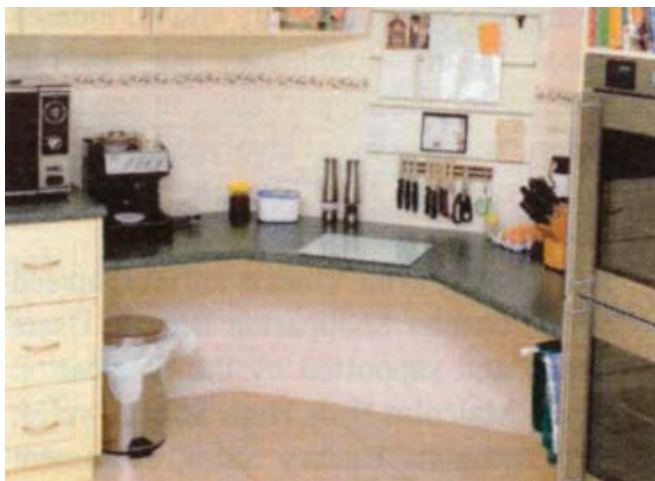
The use of more drawers and a lowered bench make food preparation easier
